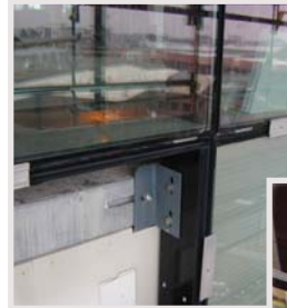
Curtain wall cladding fixed on anchor channels on the edge of slab
