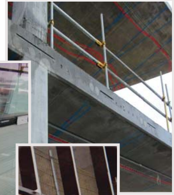
Curtain wall cladding fixed on anchor channels on the edge of slab
