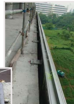
Curtain wall cladding fixed on anchor channels on the top of slab
