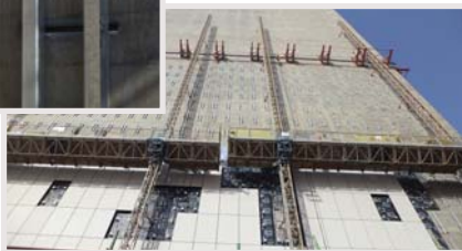
Stone cladding on secondary structure fixed on anchor channels
