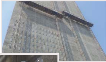
Stone cladding on secondary structure fixed on anchor channels
